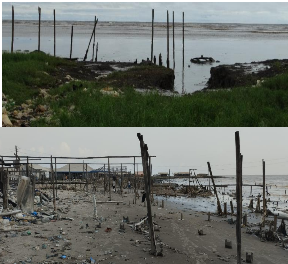
Figure 7: Destruction of Biodiversity and Infrastructure in Ilaje Coastal Area by Ocean surge
