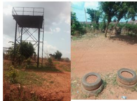
Plate 2: Poor condition of the water facilities in Alagbaka (Investment) Police Barrack, Akure
