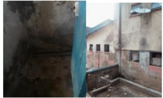
Plate 3: Interior and exterior views of toilet facilities in police barrack, Ibara Abeokuta Source: Author's Survey, 2026
